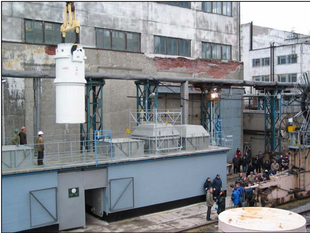
Fig. 3. The TUK-108 Prototype Container (without fuel) being placed in the Storage Facility during the November 2003 Project “Promotional Event” noting the completion of the Facility construction.
