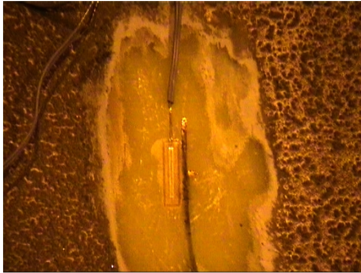
Figure 2.1 Strain gauge mounted on the weather-side of panel G
